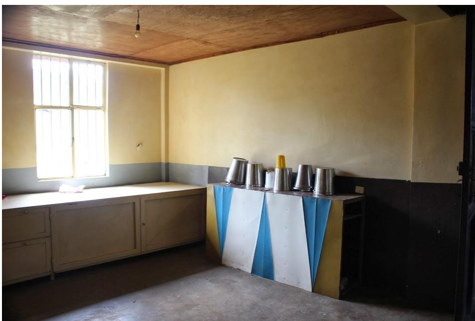
Milkcollecting Room and future Lab, 6*8*3 meter, later on temporary expansion with milktank etc.
