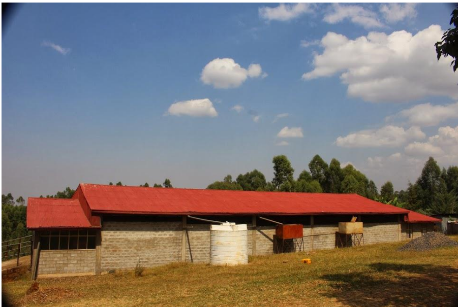
Sideview towards the tie up stable, collection of rainwater
